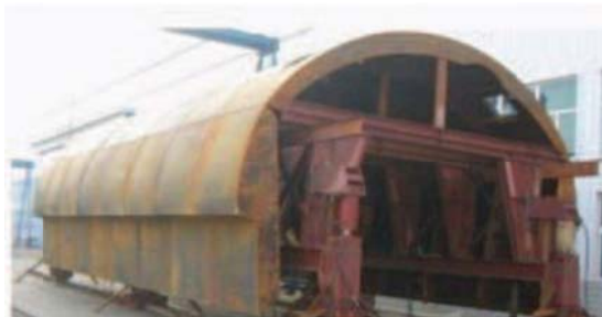
Figure 4. A view of a hydraulic frame used for the tunnel construction.
